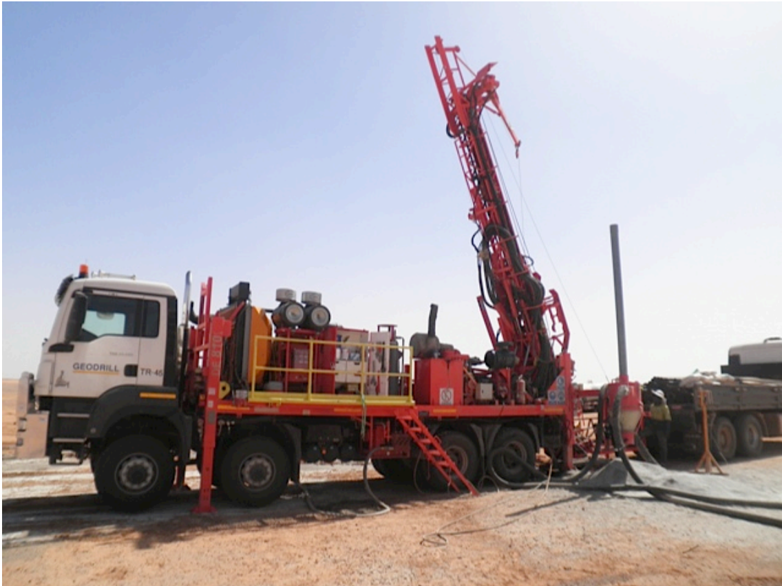
GeoDrill geotechnical inclined drilling currently underway November 2
