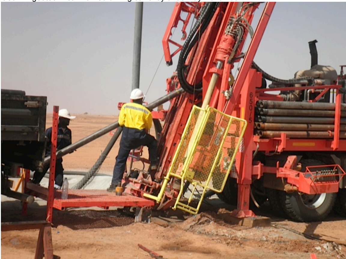
GeoDrill geotechnical drilling crew – rod change underway in November 2012
